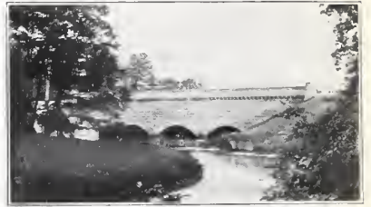
GORDON PARK AQUEDUCT Carry Intercepting Sewer, Twelve Feet, Nine Inches in Diameter
